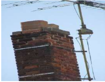
Missing chimney cap
