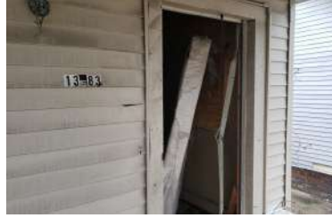
Missing door, damaged frame
