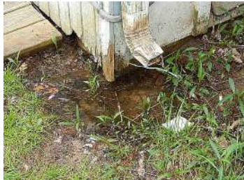
Pooling water near foundation
