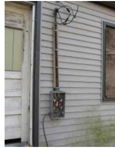
Exposed conductor
