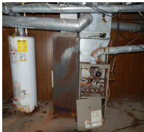
Water damaged furnace and water heater
