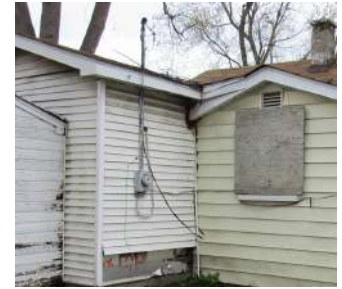
Exposed wires
