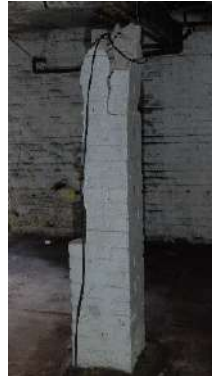
Failed brick column
