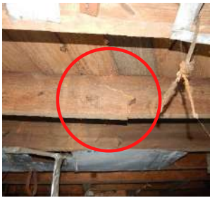
Cracked joist
