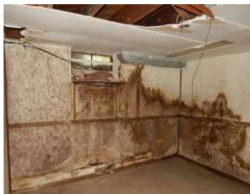
Evidence of water intrusion
