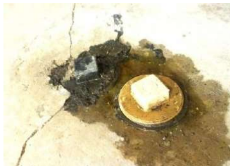
Leaking clean out plug
