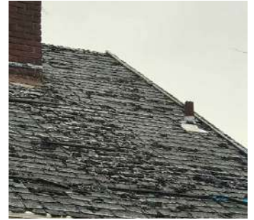
Deteriorated shingles
