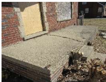
Cracked porch deck
