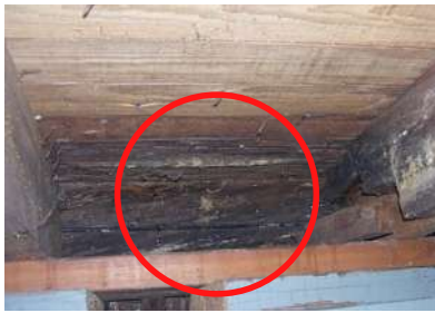
Rotted subflooring and joist
