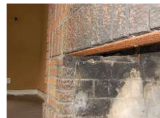
Damaged firebrick
