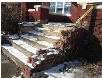
Collapsing porch wing wall
