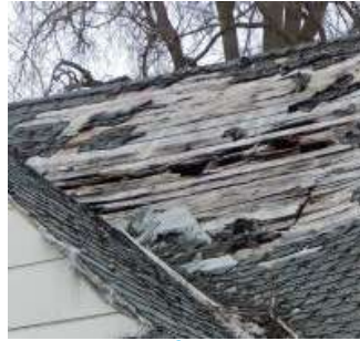
Exposed roof deck
