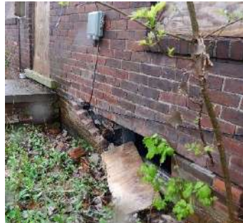
Failed exterior brick wall
