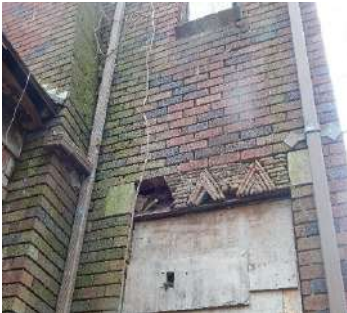
Missing brick above lintel
