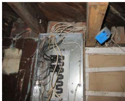
Cut and missing wiring
