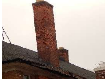
Open mortar joints
