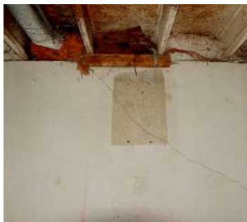
Cracked poured foundation
