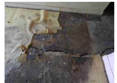
Cracked slab foundation
